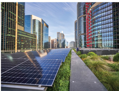
Solar panels integrated with green roof on Daramu House, Gadigal Land (Image: Lendlease)
